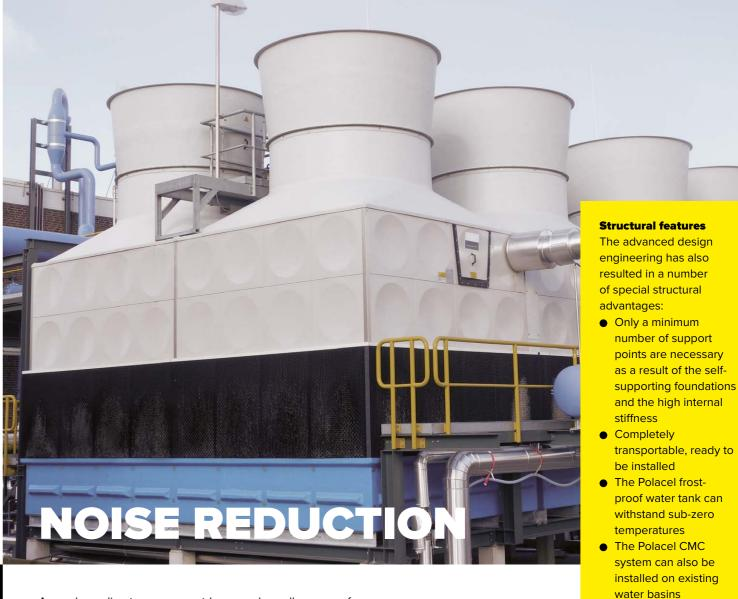
at the edge of the site. The noise produced by the cooling tower caused by, among other things, the fan, falling water, the electrical motor or geared motor, can therefore present a problem.
